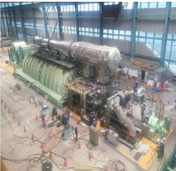
1000MW Turbine Maintenance
